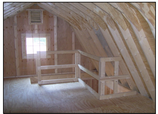
RAILING FOR STAIRS
